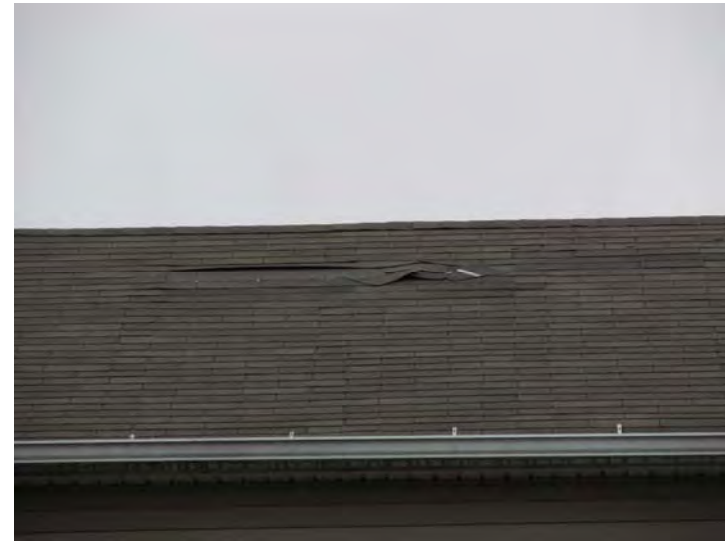
Isolated area of roof shingle damage noted on easterly side of building – Repair in near-term; replace all shingles in future
