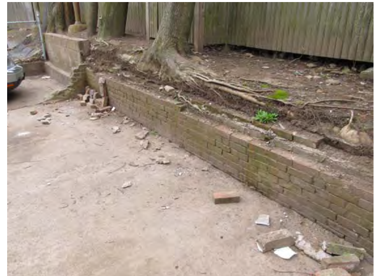
Retaining walls at parking area are in need of reconstruction
