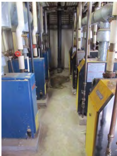
Individual natural gas-fired boilers produce hydronic heat for each unit
