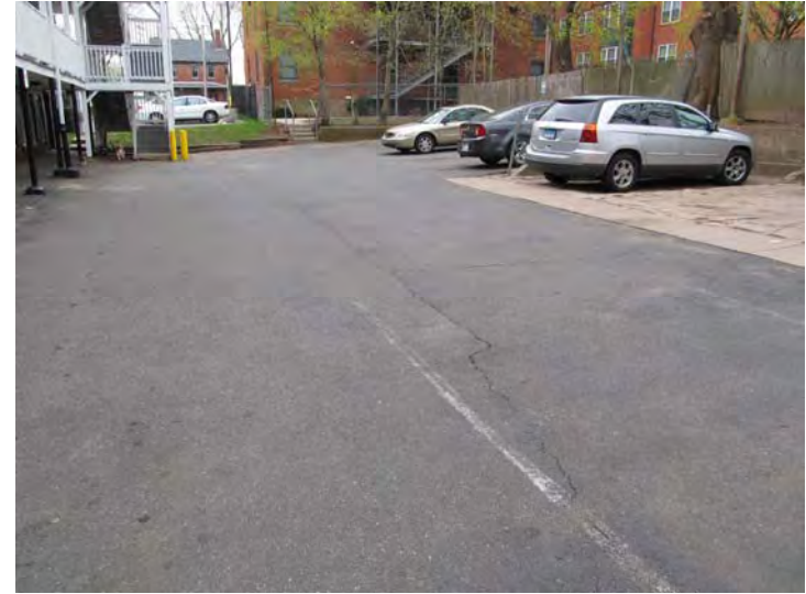
Asphalt paving at parking area is in fair condition
