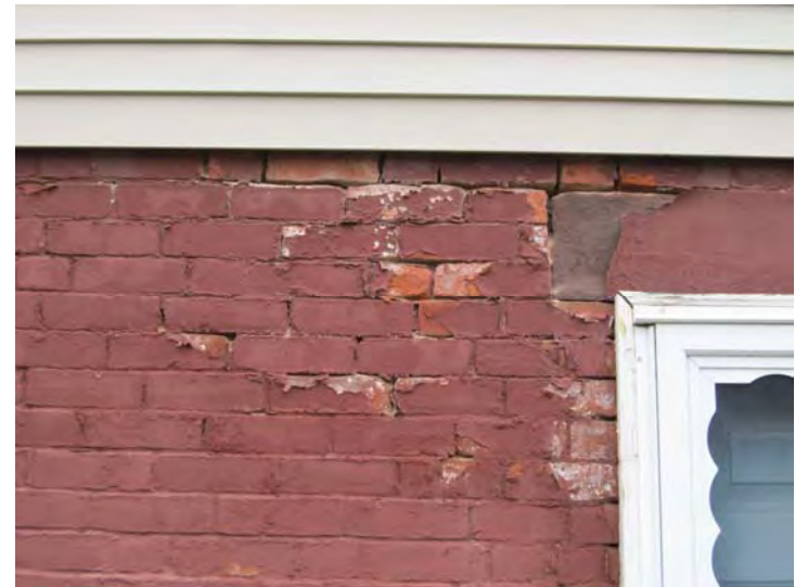
Mortar loss in brickwork also noted at various locations
