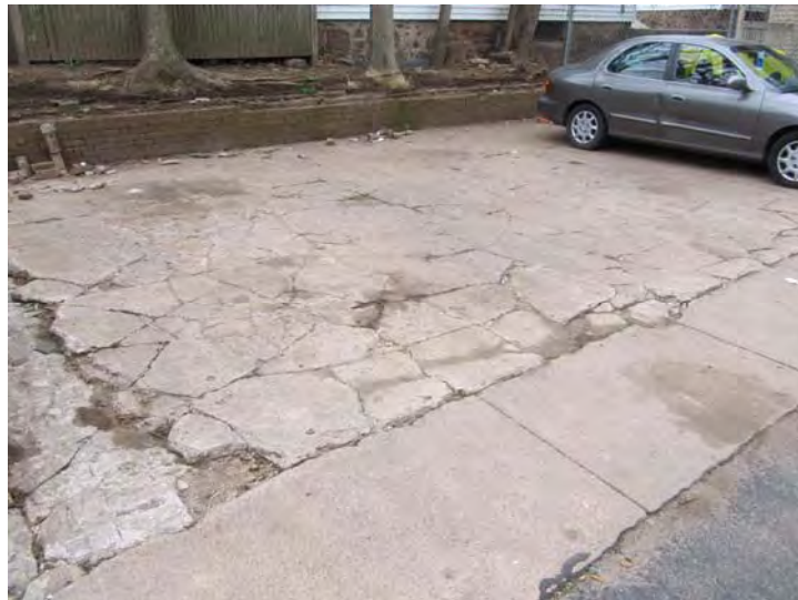
Concrete parking area surfaces are in poor condition
