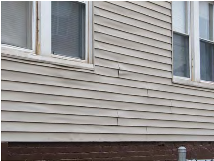
Vinyl siding varies in condition – Undulation noted at southerly elevation
