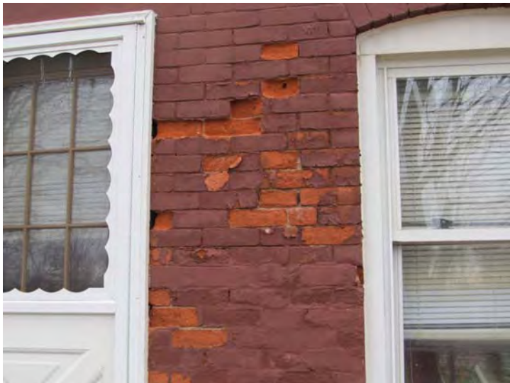
Brickwork at first floor level exhibits significant wear/deterioration at some locations – Most prevalent at rear elevation
