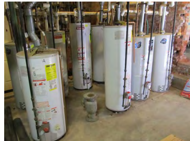
Freestanding tanks of varying ages serve the units' domestic hot water generation needs
