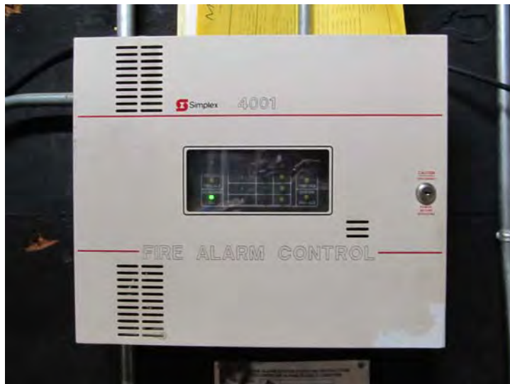
Original fire alarm control panel is serviceable but beyond its expected useful service life
